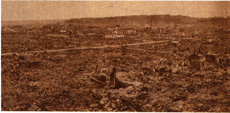
The ruins of downtown Yokohama after the Great Kantō Earthquake of 1923.(From the
